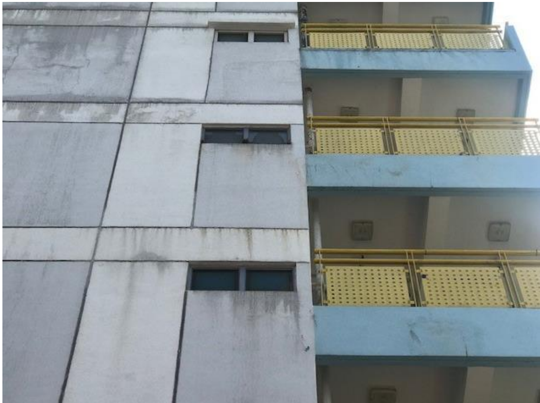
4/F & 5/F External Condition
