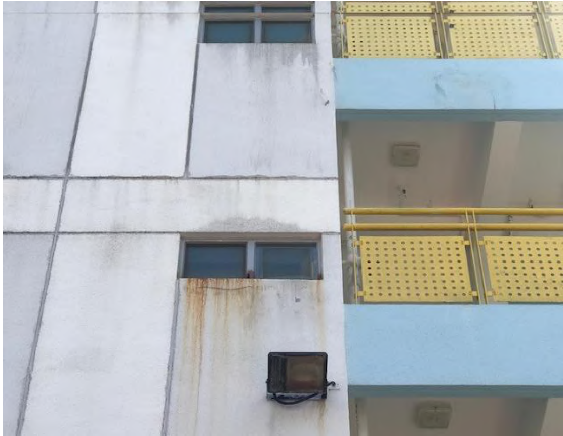
3/F External Condition
